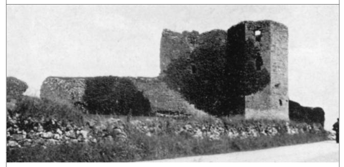
Bottom: View of Southwest corner tower by unknown photographer, published by Fitzpatrick in 1935. Note the base batter has been repaired. The ivy growth that now covers much of the stonework is already established but it is possible to make out details on the residential block, while the fabric of the west perimeter wall north of the tower is exposed.
