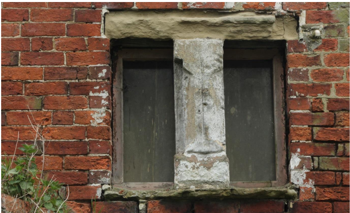
Figure 25 Window head reused as a mullion in Building 8 (Ex Situ Feature Number 001), looking east
