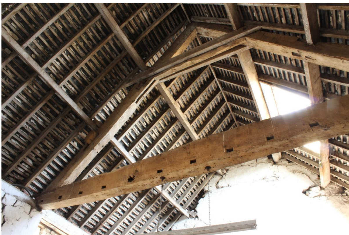
Figure 37 Reused timbers in Principal Truss 3, Building 5 (Ex Situ Feature Number 012), looking north
