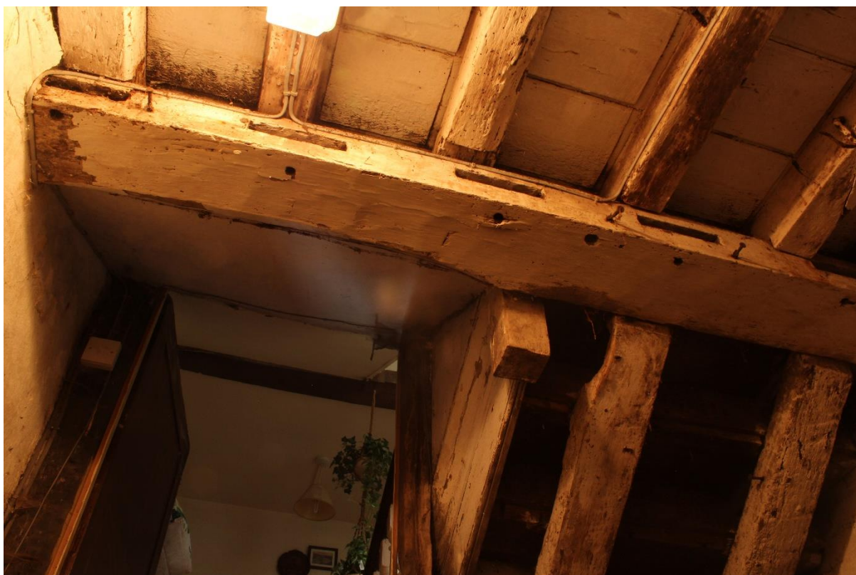
Figure 57 Reused timber incorporated into the underside of the farmhouse stair, looking south
