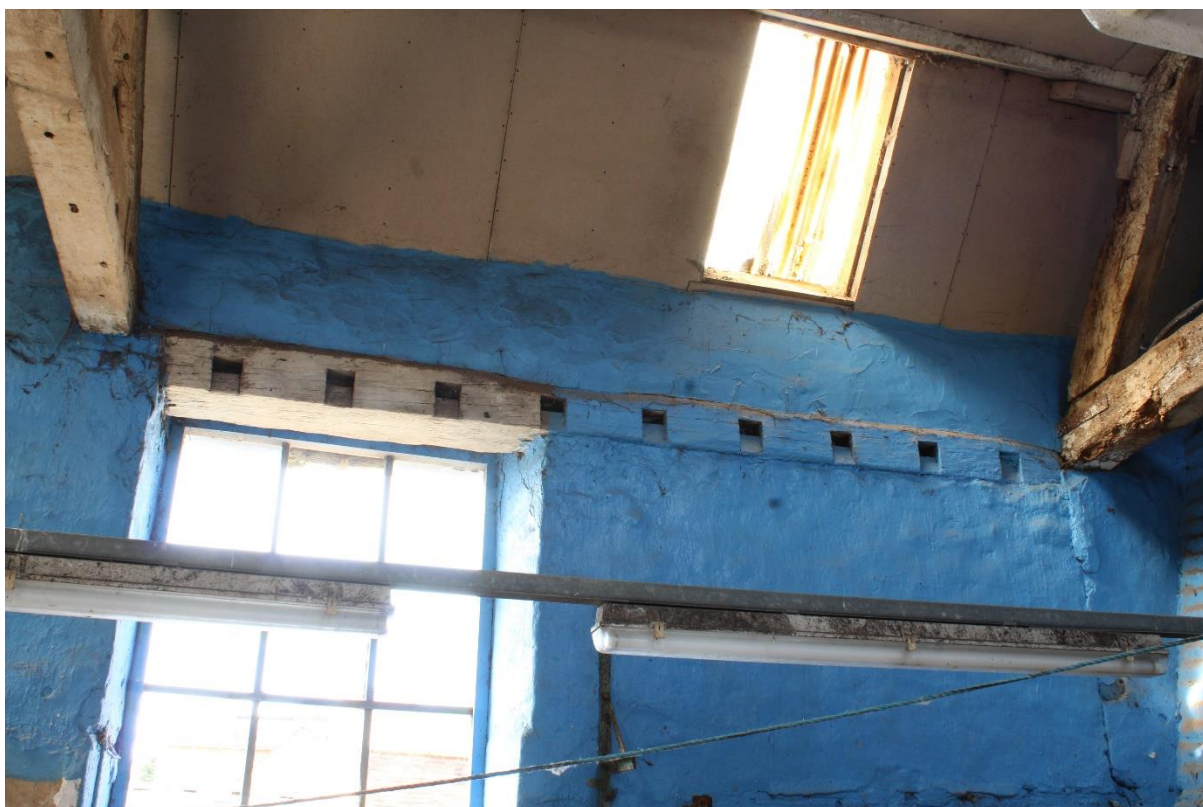
Figure 34 Floor beam reused as a window lintel in Building 5 (Ex Situ Feature Number 010), looking west
