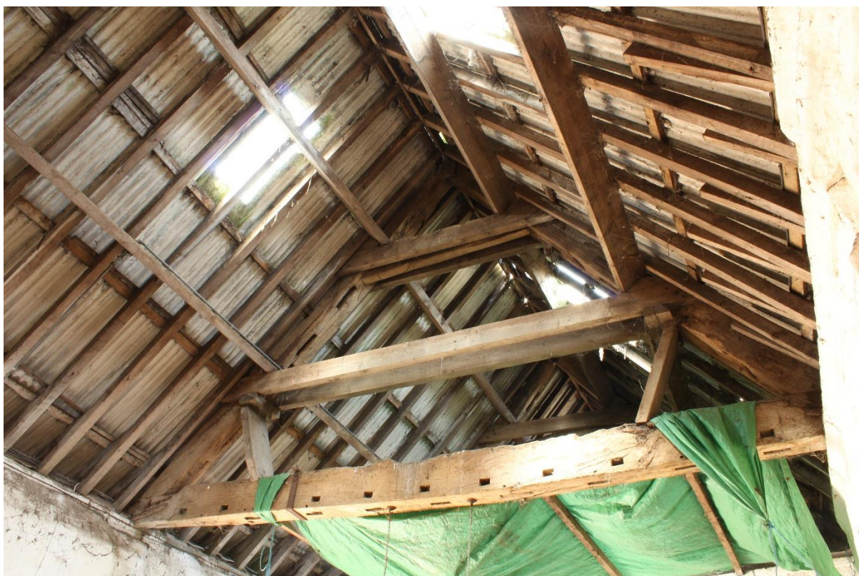
Figure 38 Reused timbers in Principal Truss 4, Building 5 (Ex Situ Feature Number 013), looking north
