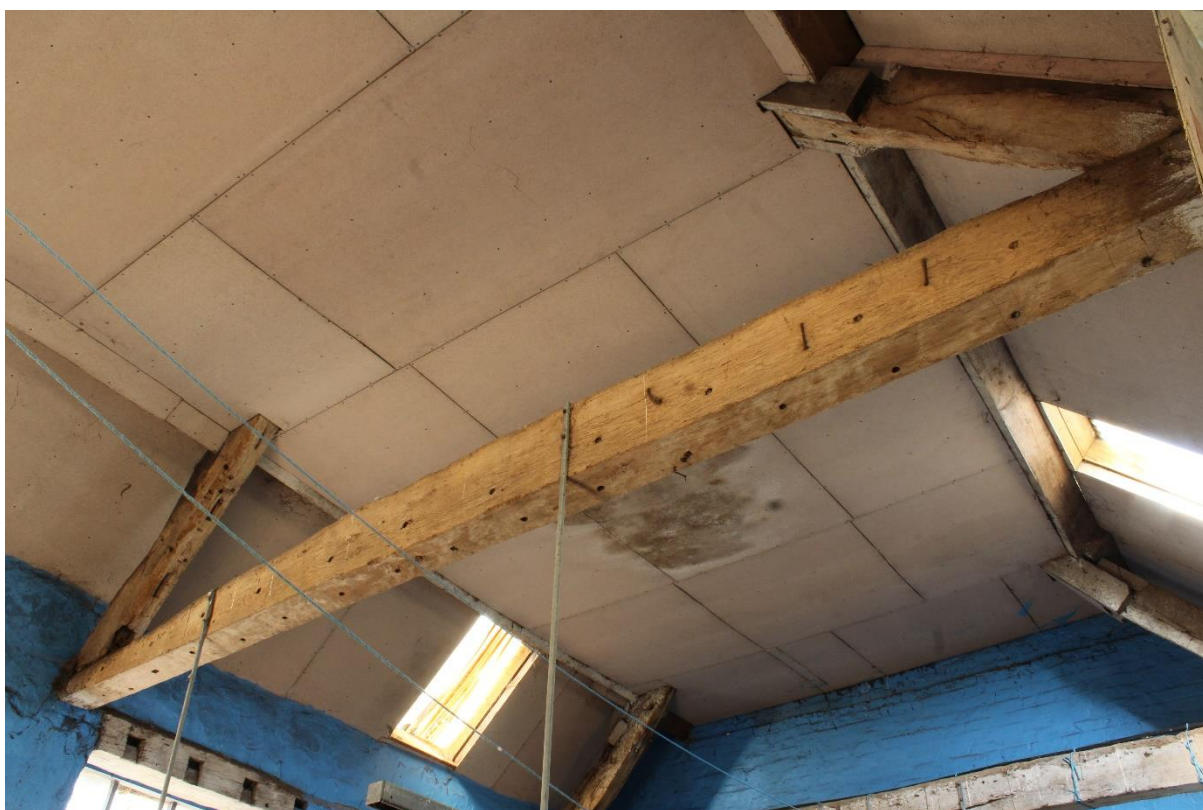
Figure 35 Reused timbers in Principal Truss 1, Building 5 (Ex Situ Feature Number 011), looking north-west
