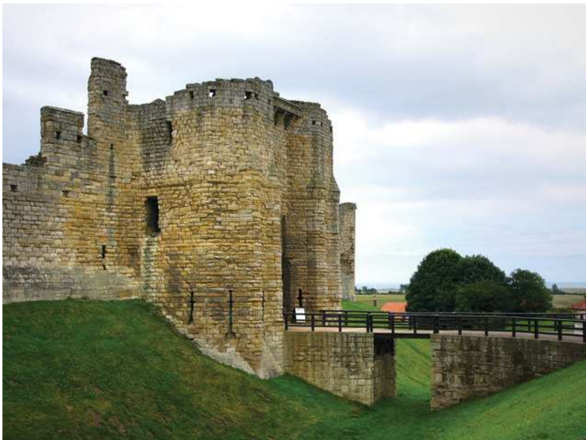
Figure 5. Gatehouse of Warkworth Castle, looking east. Chris Gunns / Warkworth Castle, entrance / CC BY-SA 2.0.
