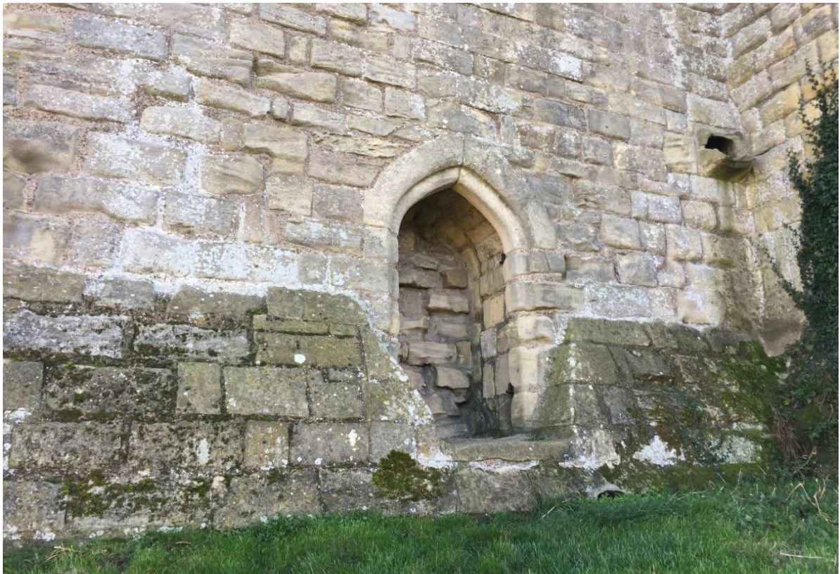
Figure 9. Photograph of the postern within the Great Tower, giving access to the motte-top area outside the embrace of the curtain walls, in the north-west of the ground floor. Note the door threshold is seamless with the floor level of the passage inside, for ease of use. © William Wyeth
