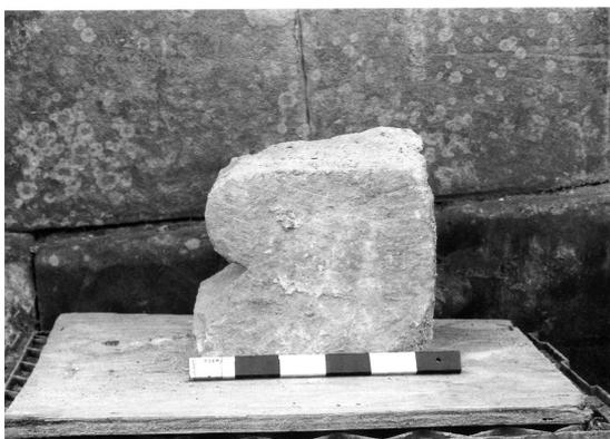
Comparable to simpler corbels for crenellations, but much smaller and with a fillet at the outer face, a refinement. Would therefore likelier have supported a projecting feature like a niche rather than supporting main parapets. However, note that its fillet is similar to the early C17 moulding (NFW 12), raising the possibility that it may be castellar revivalism.
