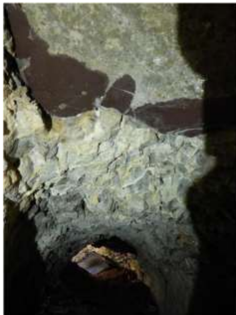
43c: roof vault, and concrete replacement slab, facing north towards entry.
