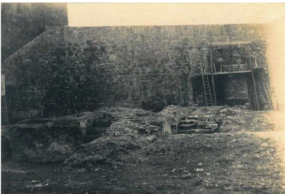
Figure 56: Outer ward: Building G under excavation in March 1931, facing due south with the Henry VII tower, recently restored, to the left. The base of a stair, probably in the south wall of the southern wing, can be seen, with a further stair to the right? (© Pembroke Castle Trust).
