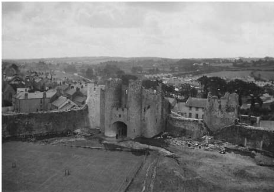
Figure 54: The outer ward in 1929, before excavation of Buildings G and H , facing southeast from the top of the keep. The northern wing of Building G is visible as a parchmark; the rest of the building lies beneath overburden (© Pembroke Castle Trust).
