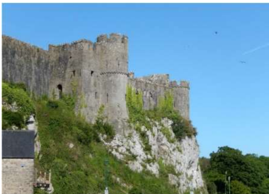
Figure 48: Outer ward: St Ann's Bastion, external façade from ESE.
