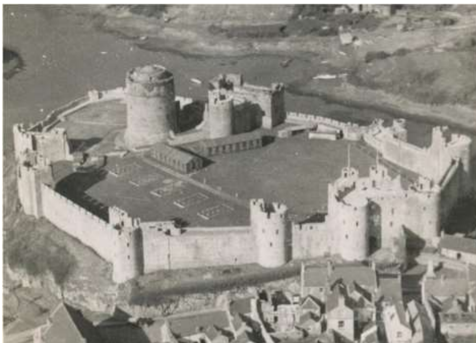
Figure 46: Undated aerial photo of Pembroke Castle during WWII, facing north, showing two long Hall Huts, and the five other huts now represented by features C . (from the collection of Adrian T. A. James)
