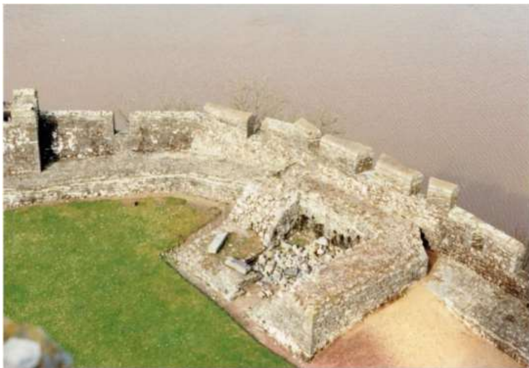
Figure 41: Inner ward: the North Turret, facing northwest, taken from the top of the keep in 1987 before the rubble was removed from the interior.
