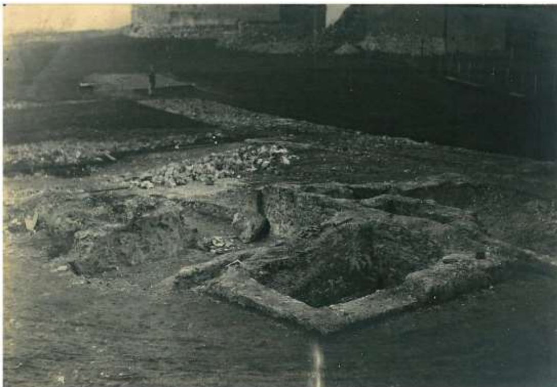
Figure 55: Outer ward: Building G under excavation in March 1931, facing WNW with the keep in the background. The large, deep chamber in the foreground is probably the cesspit mentioned in 1931. The make-up for the modern path can be seen beyond (© Pembroke Castle Trust).
