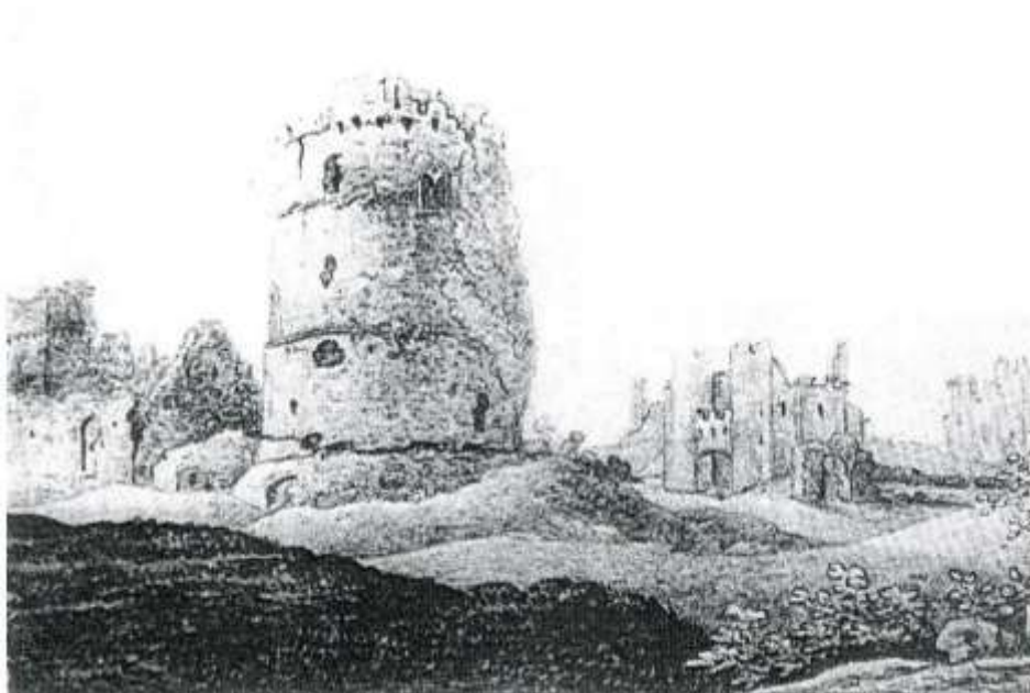
Figure 60: View of the interior of Pembroke Castle in 1802, by Sir Richard Colt Hoare, facing southeast towards the gatehouse with the keep on the left; Henry VII Tower to far right. The ruined doorway standing in front of the gatehouse must belong to Building G .
