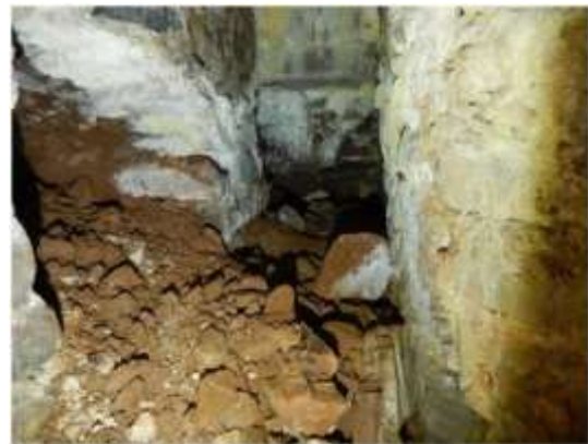
43b: side wall showing collapse (with ditch deposits beyond), and possible end wall, facing south.
