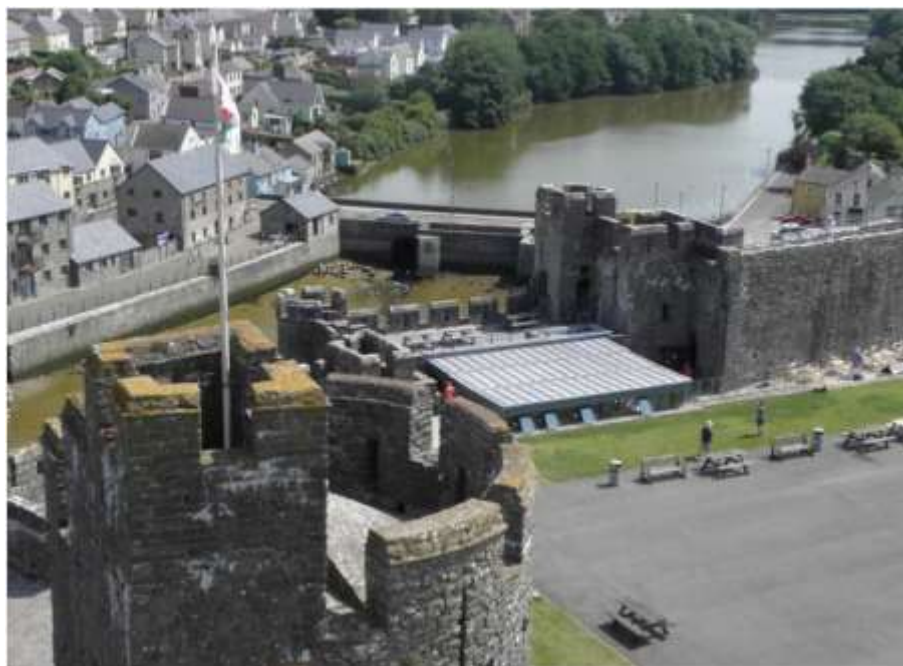
Figure 49: Outer ward: St Ann's Bastion, interior from top of keep, facing east (with the café built in 2009).
